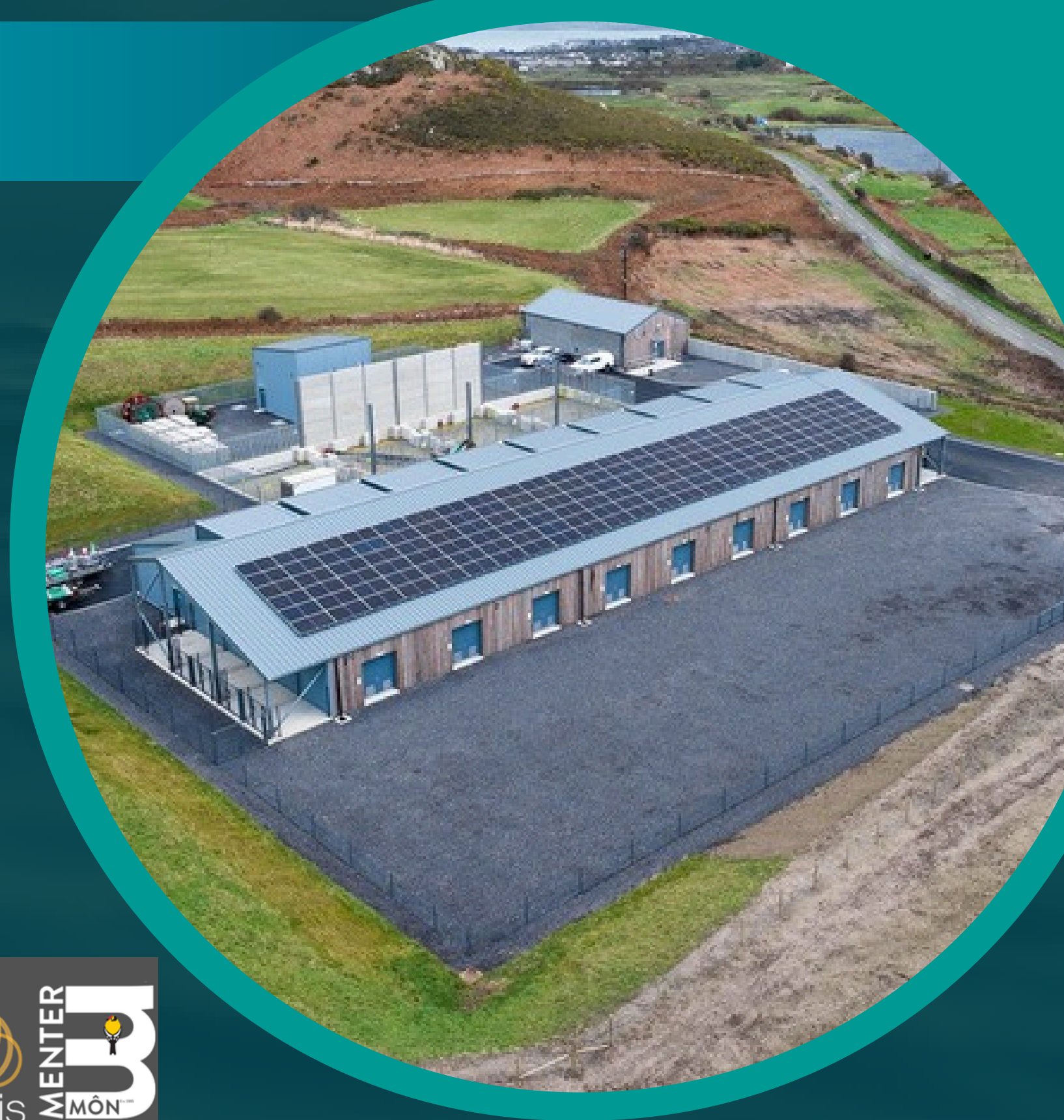
Figure 04: Morlais substation near South Stack, Anglesey, was built in 2023 after securing consent in 2021.
